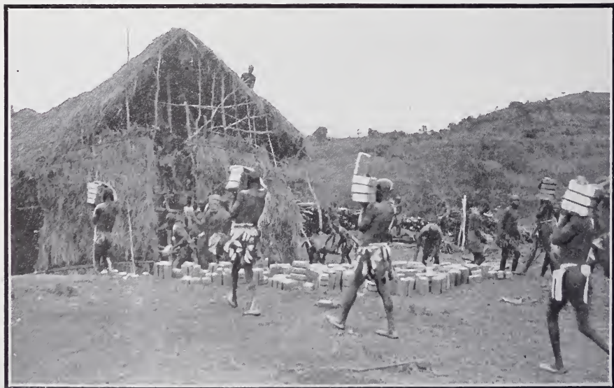
Natives carrying mud bricks to the oven or kiln in which they are seasoned before being used in hut construction.
